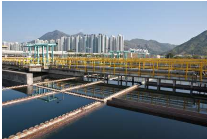
WATER TREATMENT PLANT 水处理厂
