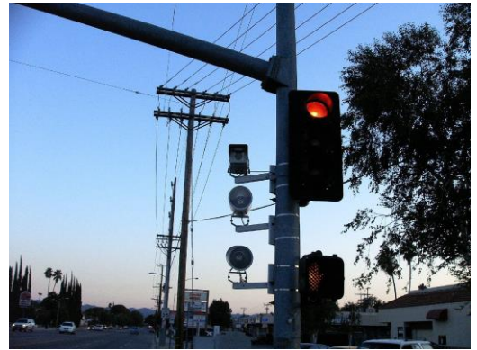
DSI-2NT-ITS TRAFFIC SIGNAL MOUNT
